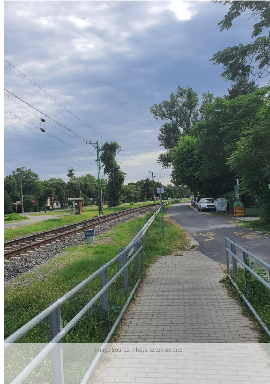
Slope leading to railway crossing - Alsóbélatelep Báthori Utcai Szabadstrand
